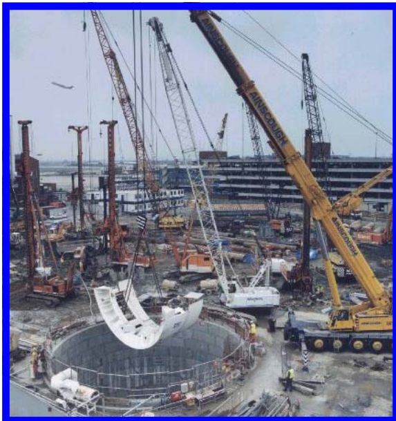
STATION SHIELD initial installation
