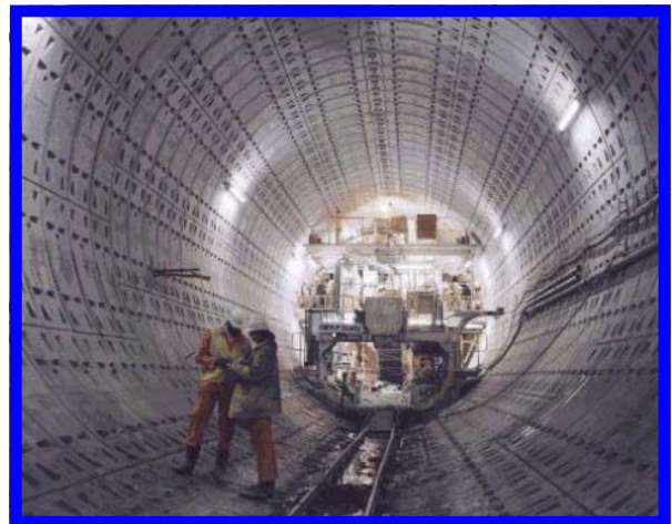
STATION SHIELD rear view in lined tunnel
