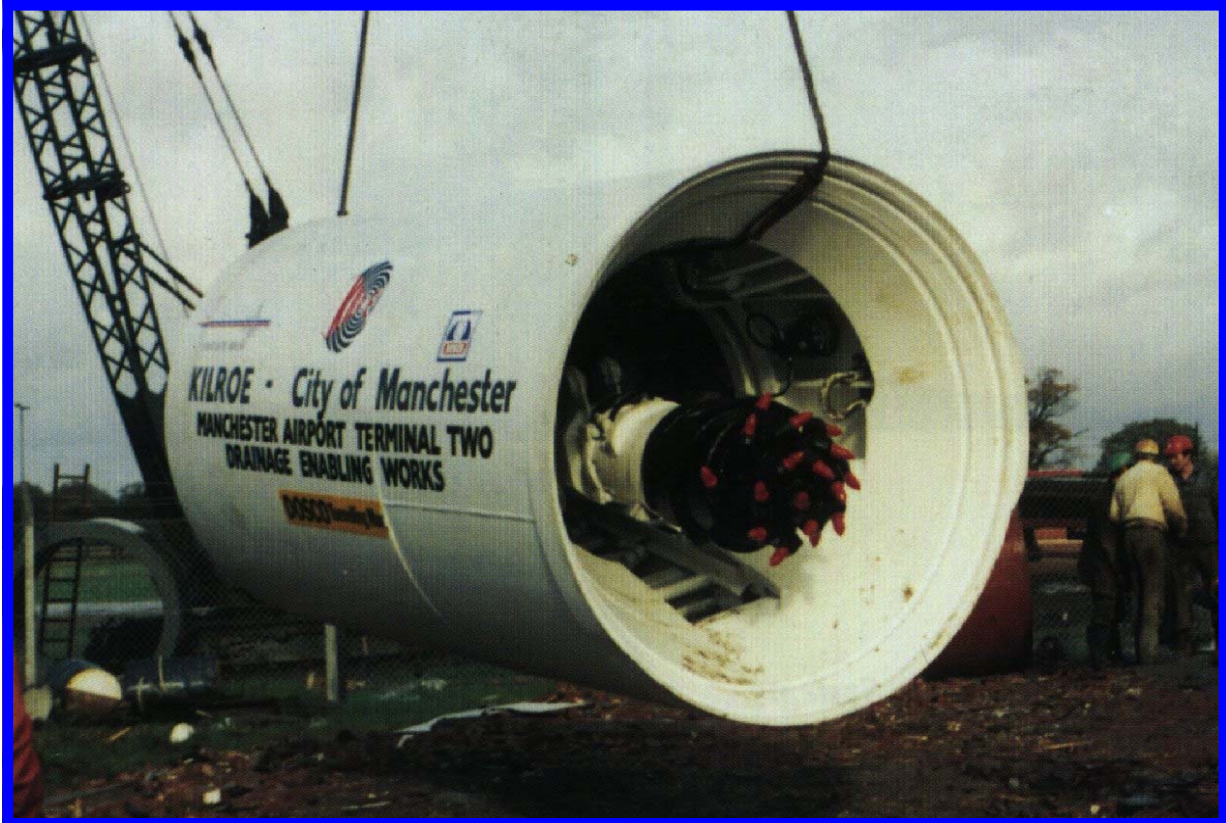
Pipe Jack machine being installed
