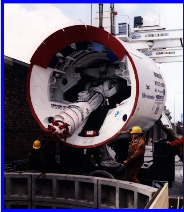
TM1800 being installed
