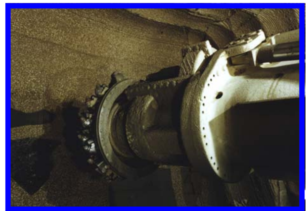
TTM100 working underground
